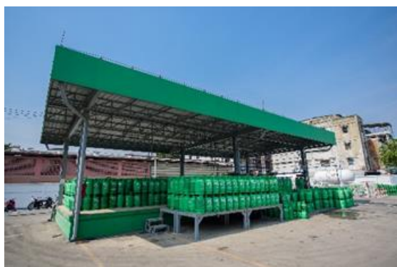
Exhibit 40: Gas filling plant
