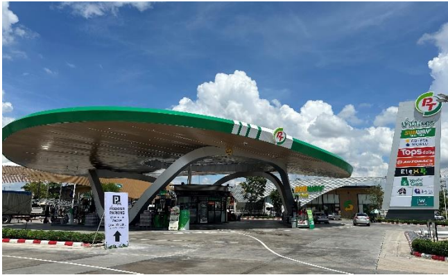
Exhibit 5: PT Max Rest station in Nakorn Pathom
